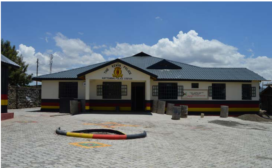
Modern Kaptembwo police station
